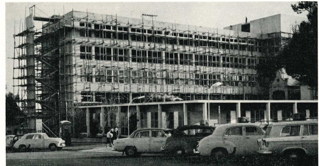
Stage One nearing completion.
