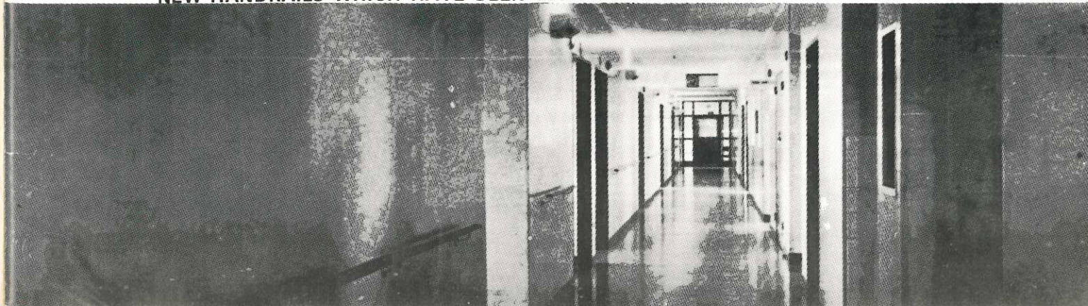
NEW HANDRAILS WHICH HAVE BEEN INSTALLED IN WARDS 1, 2 & 3.
