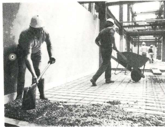
Workmen laying floor in new kitchen.
