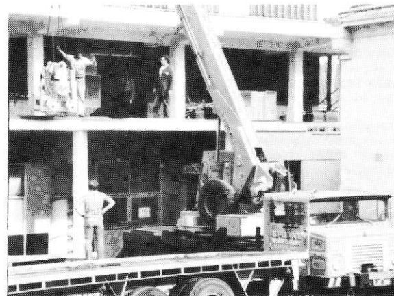
New Theatre Air Conditioning Plant being lifted to Mezzanine Level.
