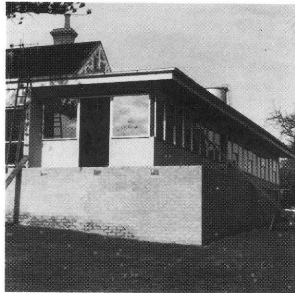
Sunroom extension under construction at Corio House.
