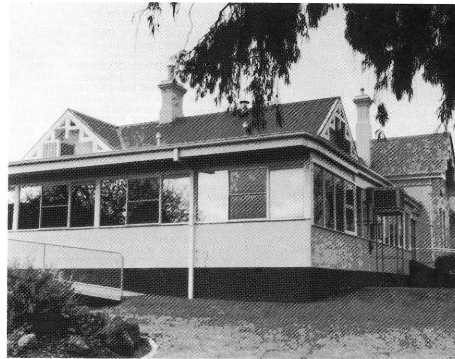
Sunroom extension at Corio.
